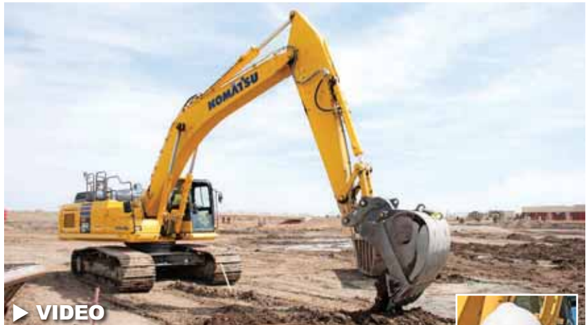
Operator Kory Lesniak digs a utility trench with a Komatsu intelligent Machine Control PC360LCi-11. "It's very accurate and smooth," said Lesniak. "You can't make a mistake. You get down to grade, and it stays right there. It can make an operator fat in no time."
