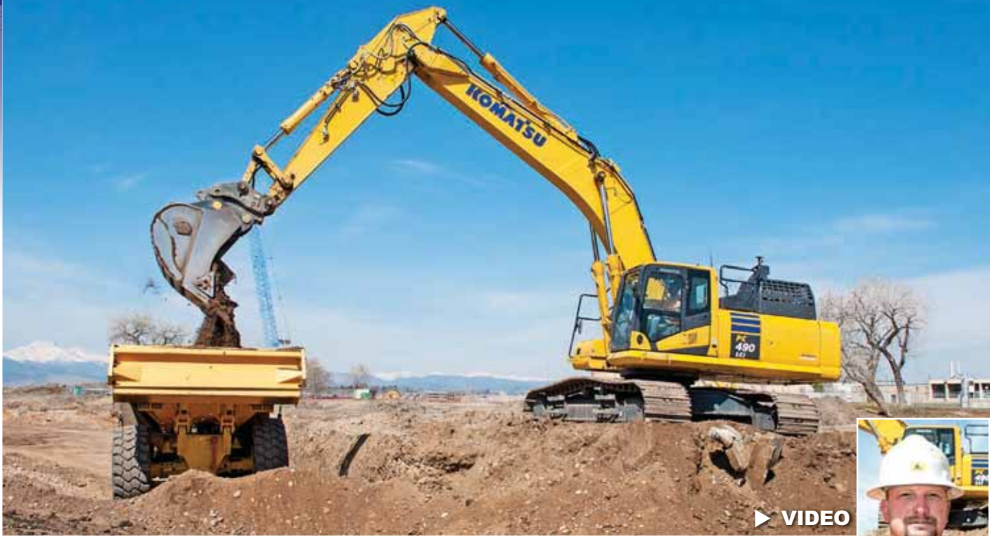
Zak Dirt Operator L.T. Snyder cuts grade and loads trucks with a PC490LCi-11 on the water park in Longmont. "I really enjoy running it," said Snyder. "The intelligent Machine Control really saves a lot of time and money. I can take four to seven feet of material out and cut grade at the same time."
