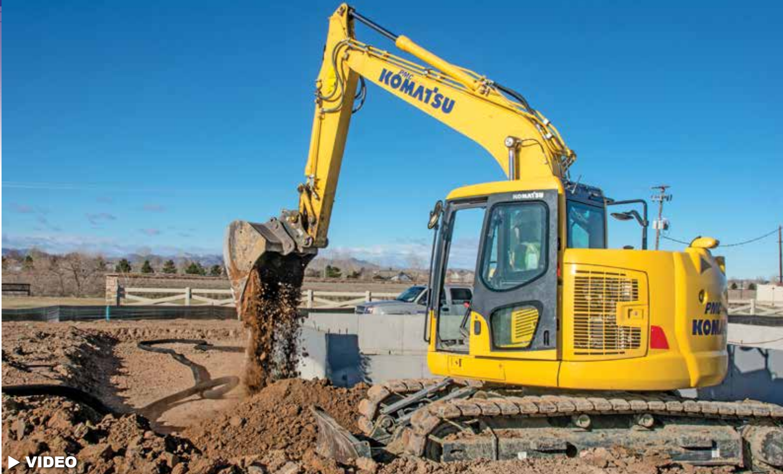
Project Foreman Levi Nicholson digs and backfills around a house foundation with a Komatsu PC138USLC excavator near Wellington, Colo. “The zero tail swing is ideal for jobsites with limited space, which is often the case on subdivisions where the houses are close together,” said Nicholson. “It’s maneuverable and powerful. Having the blade on the front assists with backfilling; it’s a great added feature.”
